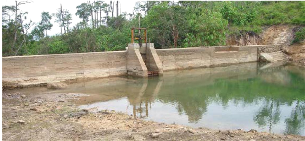
Figure 3.16 Balu Dam (in dry season), showing entry to discharge pipe and spillway
