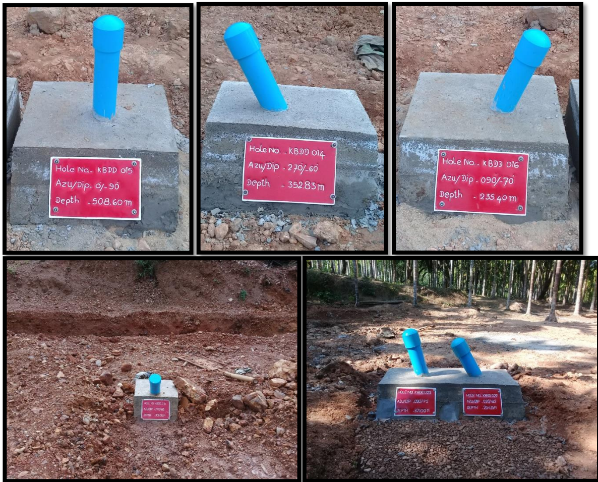
Figure 14.6 Drill hole caps
